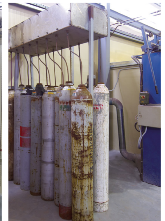
Drying Facility for Cylinders and Extinguishers, following the Hydraulic Test Procedure
