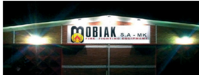
MOBIAK Balkans Distribution Center (F.Y.R.O.M)
